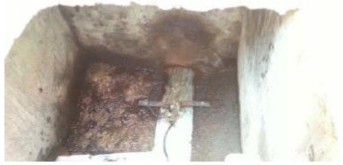
Fig. 3. Flowmeter sensor fixed to bottom of sewer pipe
